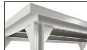
Underside supporting frame
